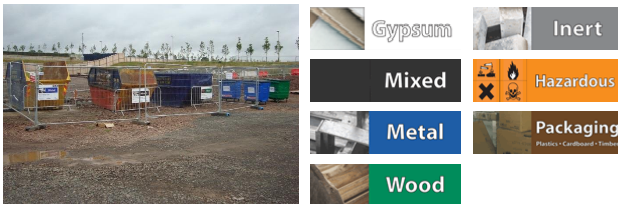
Figure 4-1 Examples of segregation skips and waste stream segregation by colour-coded signs
